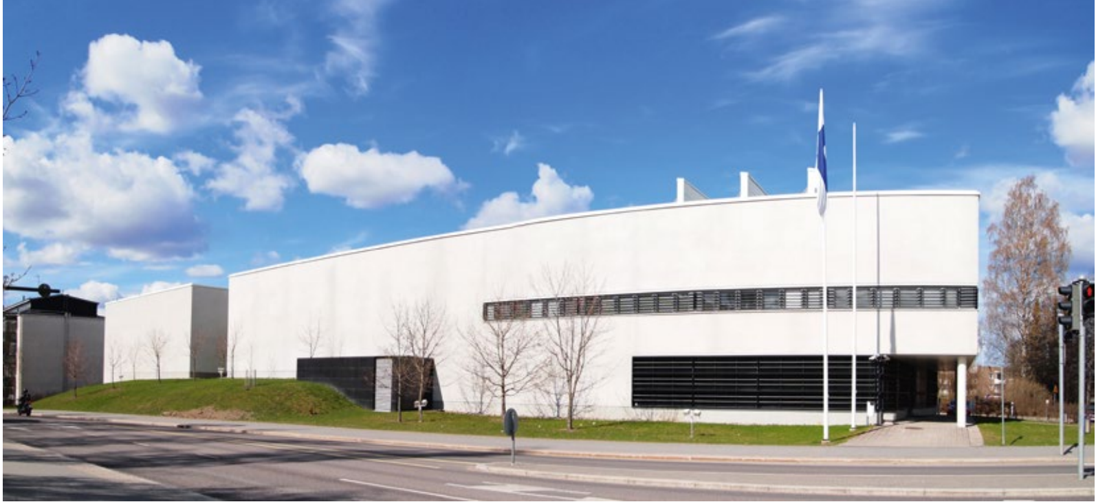
The Jyväskylä facility of the National Archives of Finland. Photo: Tiia Monto, Wikimedia Commons.
