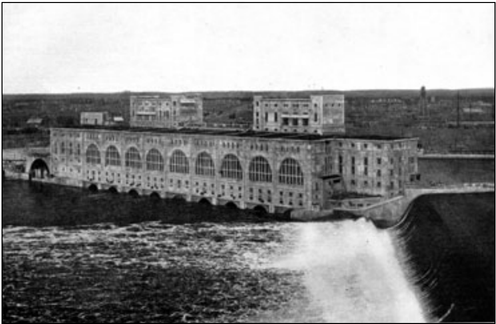
Volhovin voimalaitos. – Exterior of Volhov power station. Volhov Power Station with Sub-Station at Leningrad
